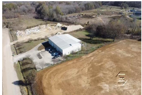
View of Subject (Photo Taken on December 1, 2020)
