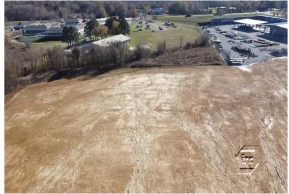
View of Subject (Photo Taken on December 1, 2020)
