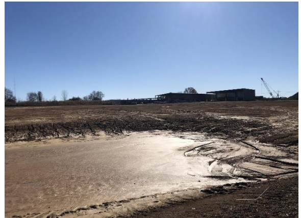
View of Subject (Photo Taken on December 1, 2020)
